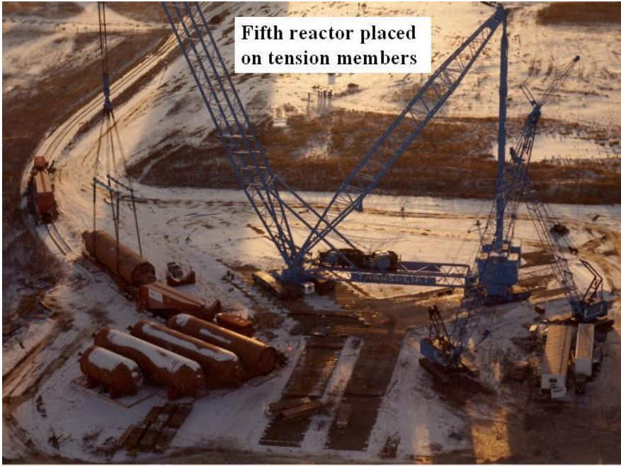
The eighth photo shows four of the reactors staged and the last one placed on the tension members.
